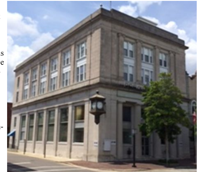
Albemarle Bank & Trust will renovate the interior of this stately building to provide for retail banking space.
